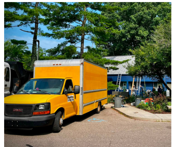
Repairs at Alpha House West have begun!
